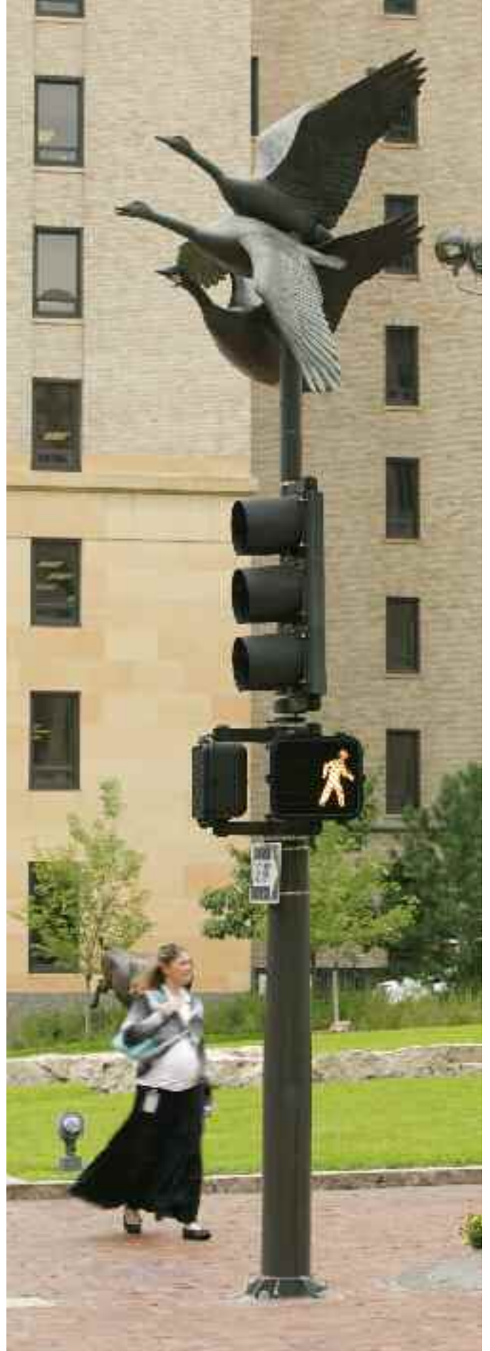
Specially designed, reinforced traffic light poles were used to bear the weight of Ullberg's bronze geese.
